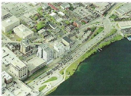
Figure 2: Aerial view of Existing John Nolen Drive
