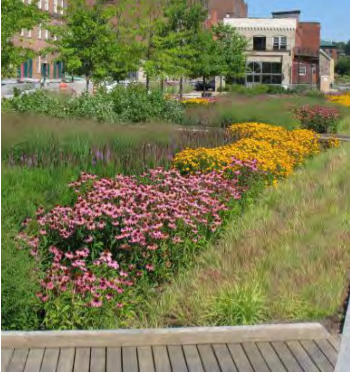
Bioswale and Rain Garden
