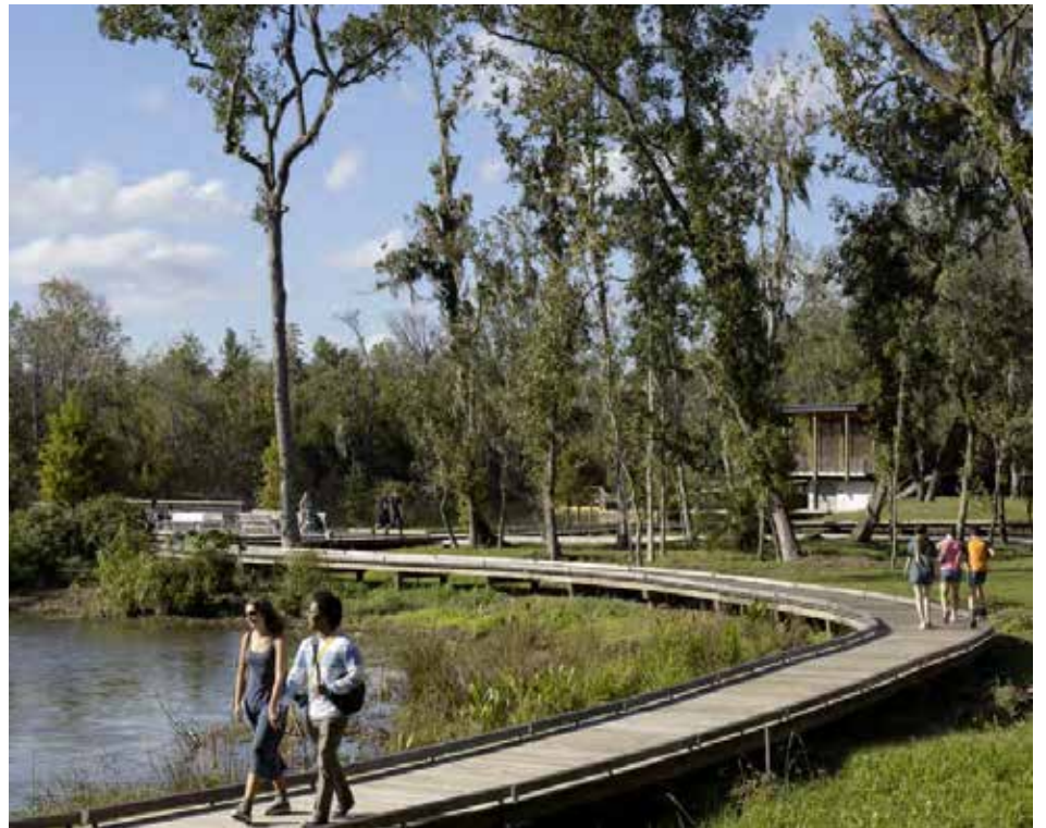
Wetland, Fish Habitat and Boardwalk
