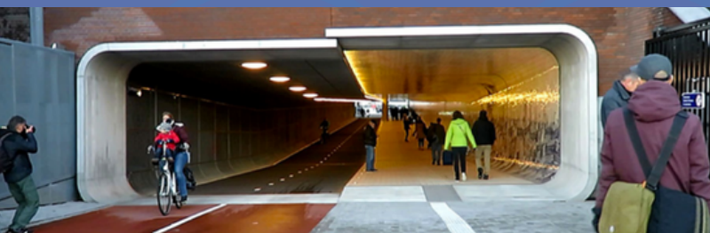
EXAMPLE OF UNDERPASS TUNNEL
